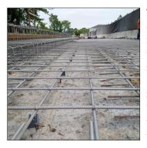
The \$4.8 million dollar rehabilitation of the Nashwaak River Bridge No.1 is included the New Brunswick government's \$409.5 million dollar investment in roads and infrastructure. Rehabilitation of the bridge was required due to minor vertical cracking in bridge piers and extensive concrete deterioration on the top mat of the bridge deck.
